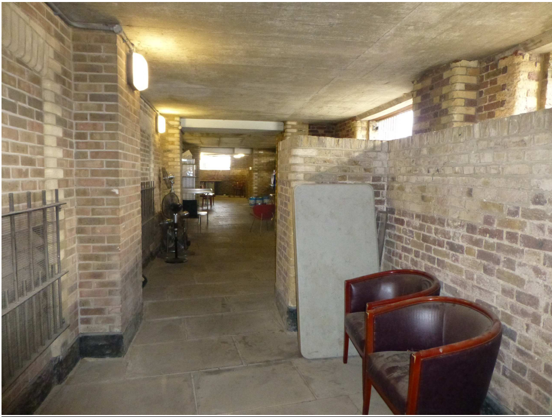
East-west section of covered walkway
